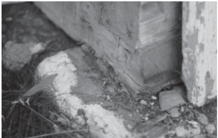
*Evidence of rot before repairs were undertaken*
